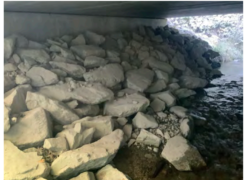
Right Bank Abutment when facing downstream
