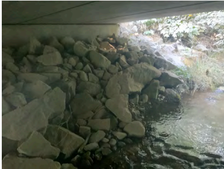
Right Bank Abutment when facing downstream
