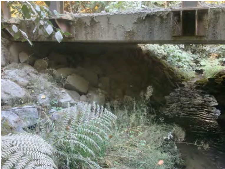
Left Bank Abutment when facing downstream
