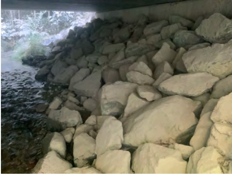
Left Bank Abutment when facing downstream
