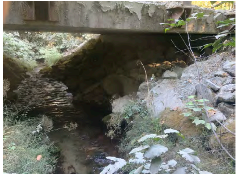
Right Bank Abutment when facing downstream
